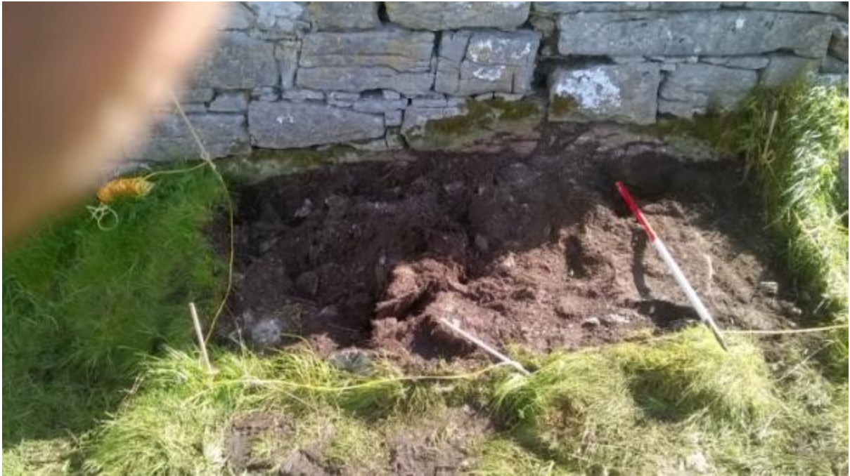
Rubble stone removed to 30cm. depth.
