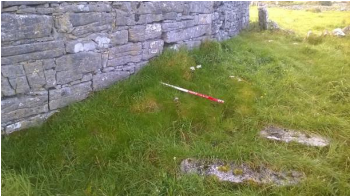
Excavation site and corbels prior to works.
