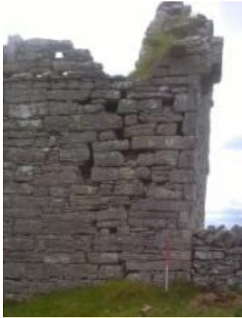
NW corner showing machicoulis and parapet.
