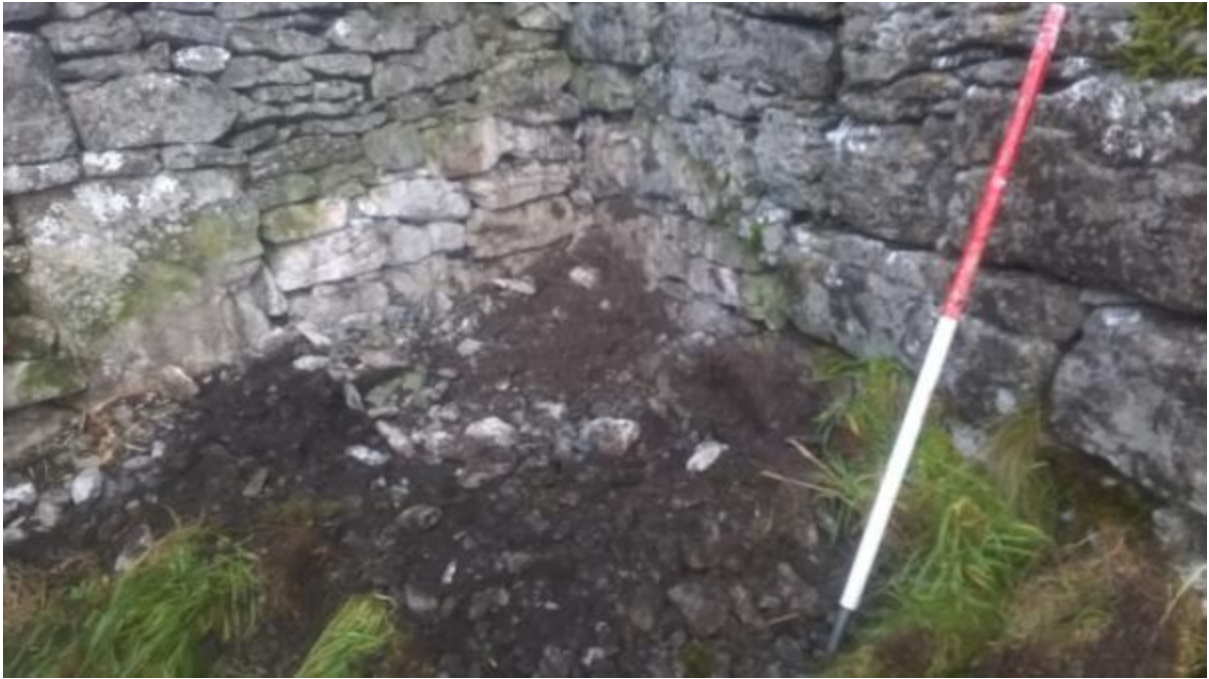
All stones removed and set aside.
