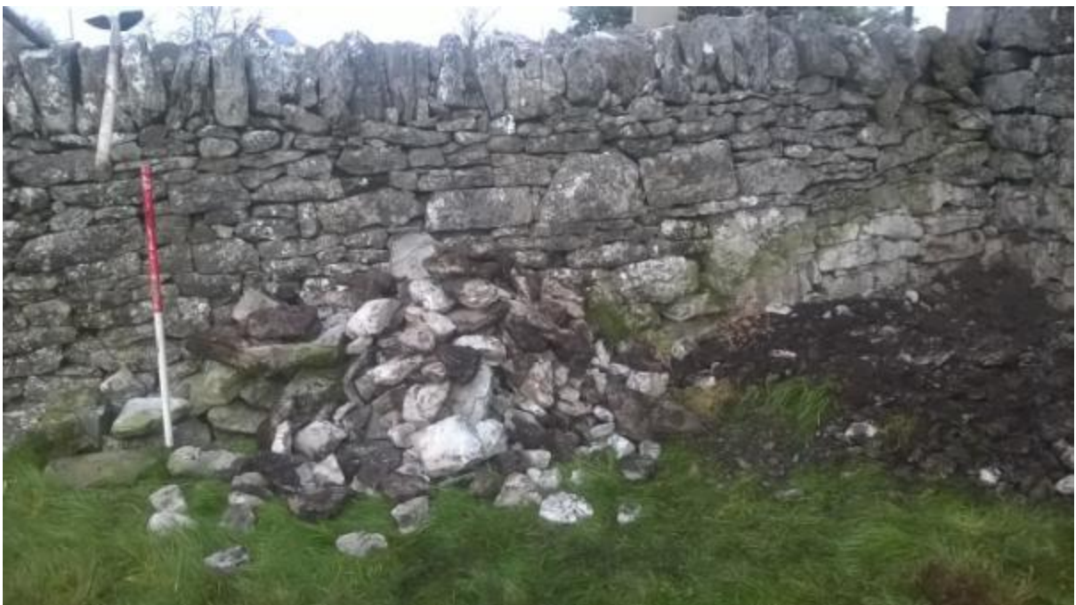
Rubble infill set aside for re-use.
