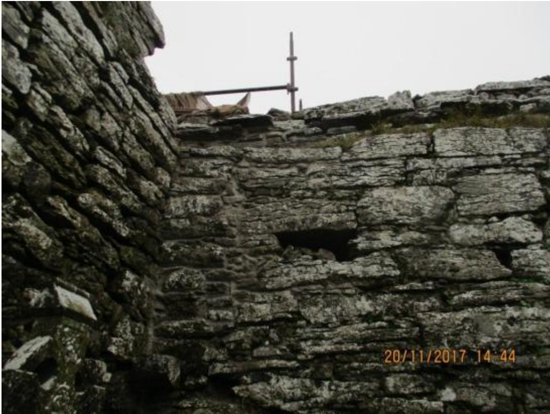
North west corner, completed (interior).
