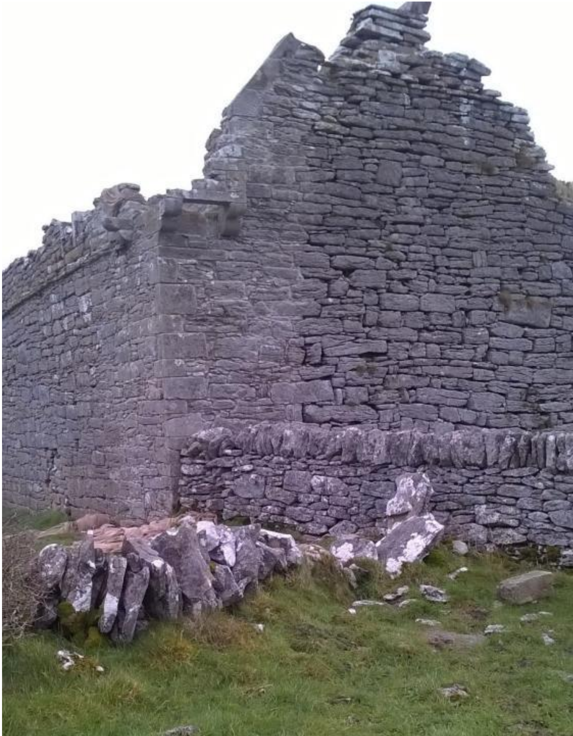
North West corner completed.
