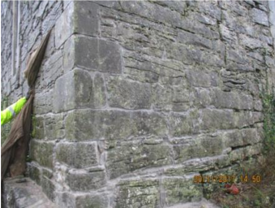
South east corner. Works completed.
