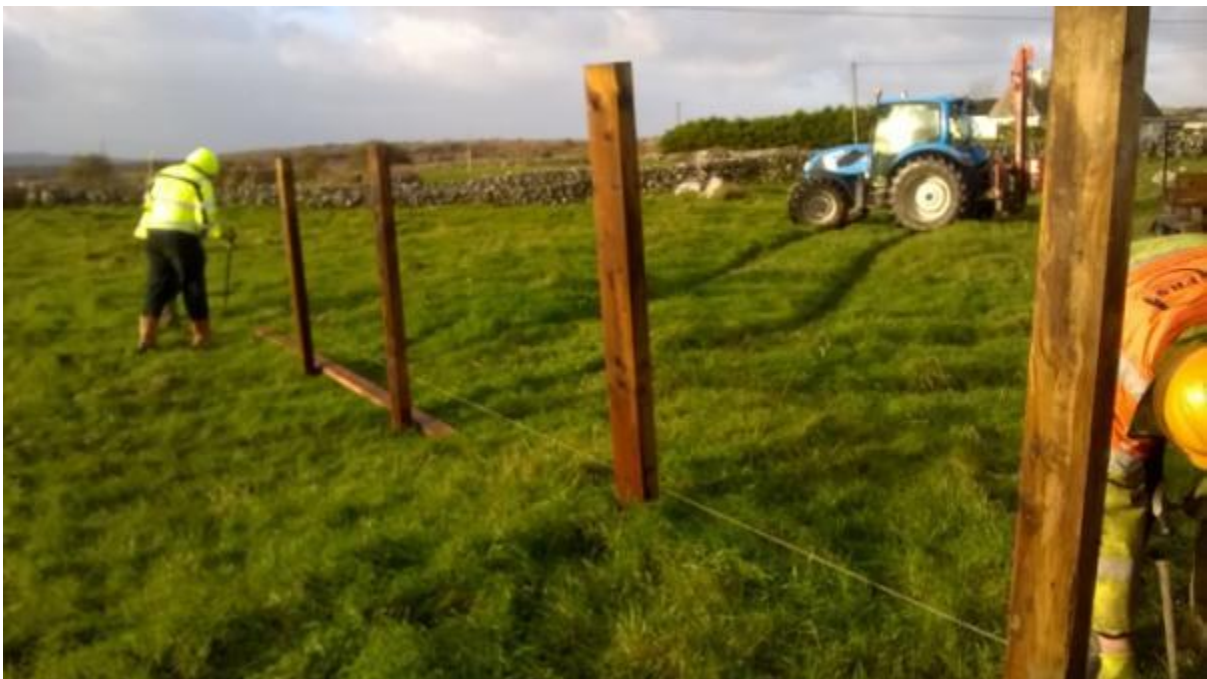
Marking out the wooden fence.
