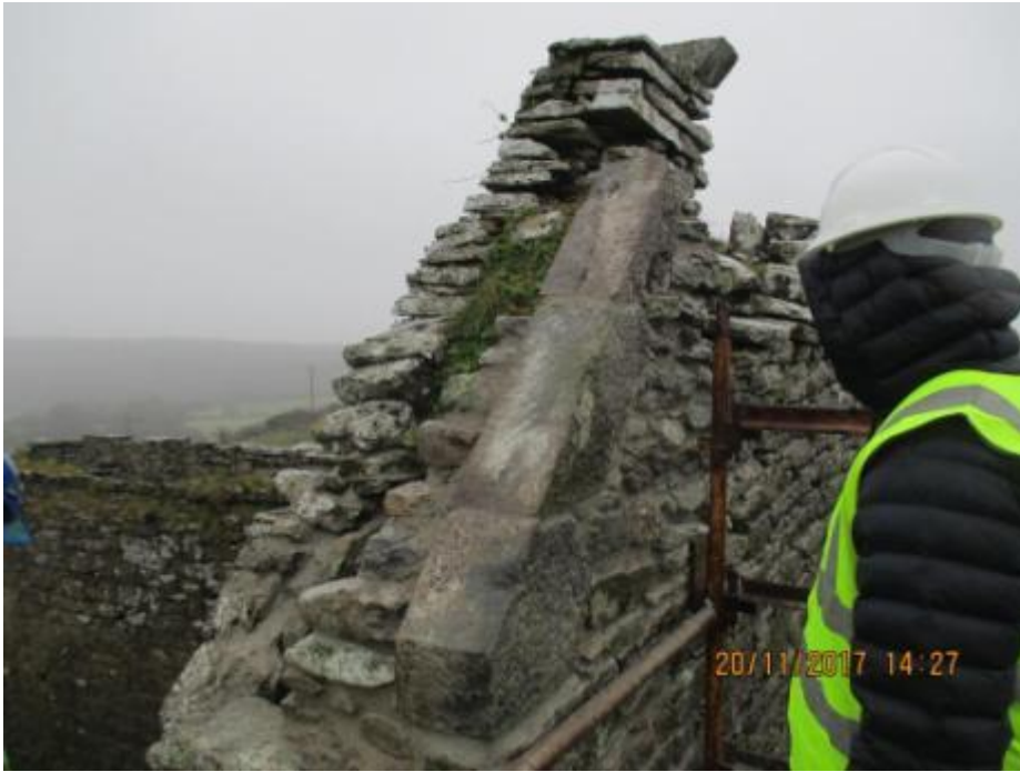
Barge stones re-instated. West Gable.
