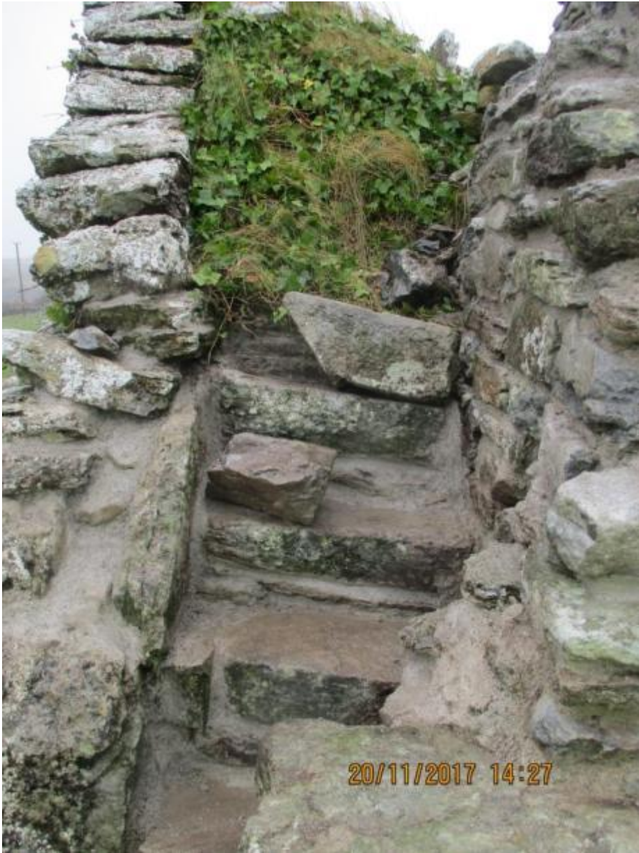
Gable steps re-pointed.
