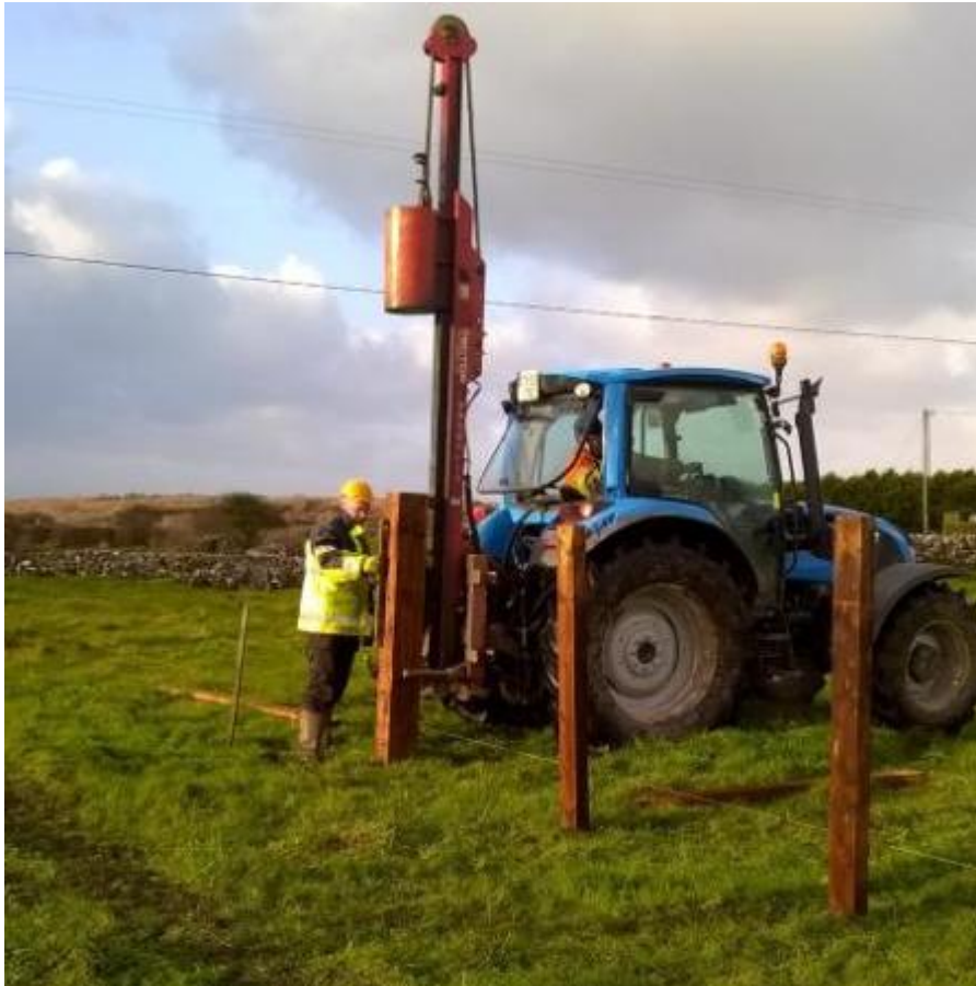
Driving the posts.
