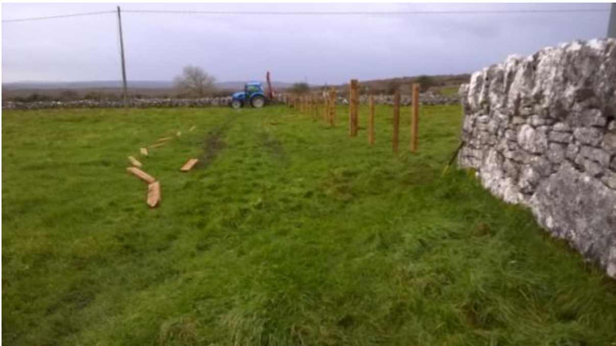
Finished north side of rail.
