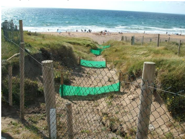
Photograph 35: Sand trap fencing along gully at north end of beach (2005)
