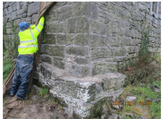
Photograph13: Corner stonework repointed
