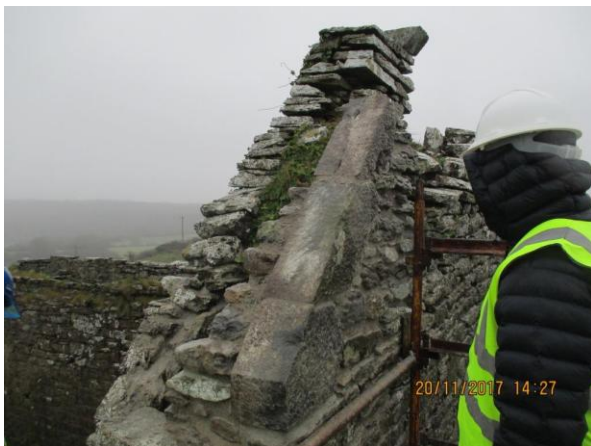
Photograph 12: Repairs to gable barge
