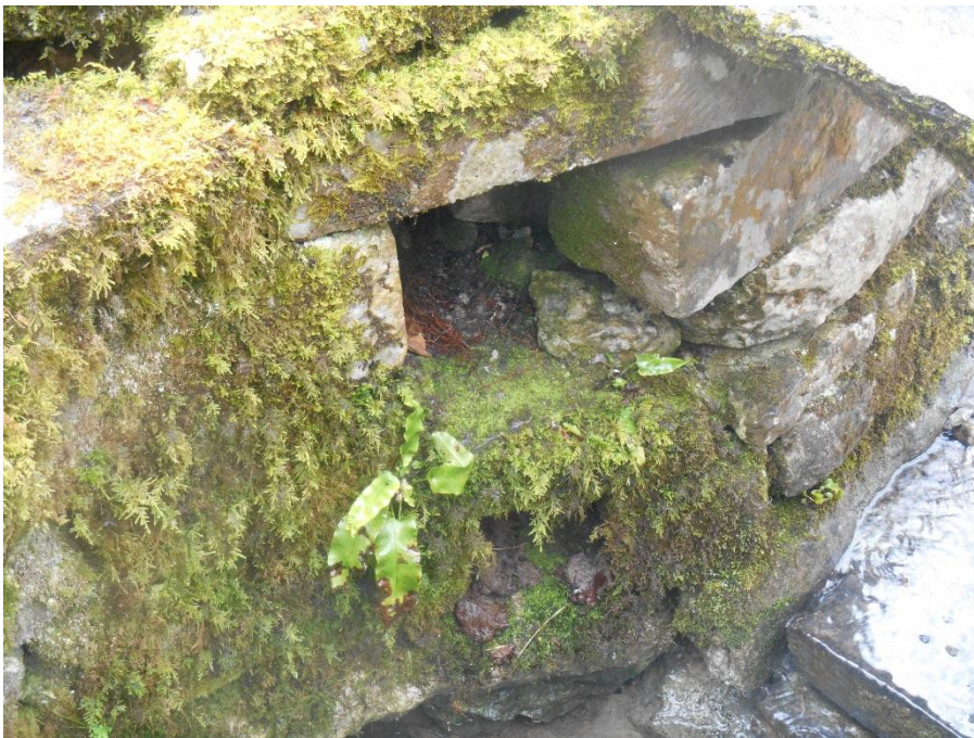
Photo 3: Possible receptacles for offerings within the well house.
