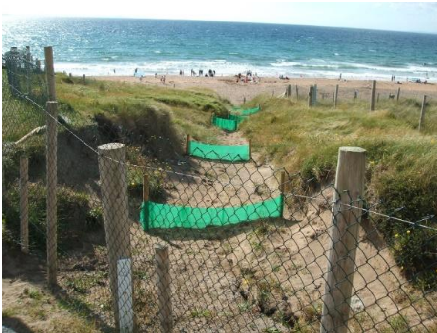
Figure 19a-b., a. Sand Trap screens with post-and-wire fencing, view north eastwards into the dune-front, Jan. 2006 (Source: AB); 19b. Sand trap Screen in eroded gully in the dune-front, northern edge of dunes, 2005 (Source: Browne, 2007). NOTE: THIS AREA OF FORMER SAND BREACHING/ EROSION HAS CURRENTLY HEALED (viz. Fig. 16a.)
