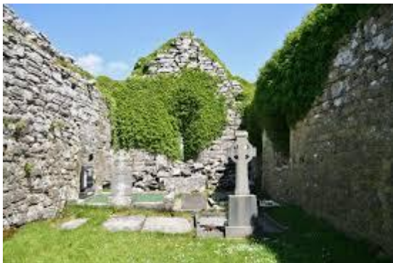
Photo 9: Ivy obscuring east window 2005
