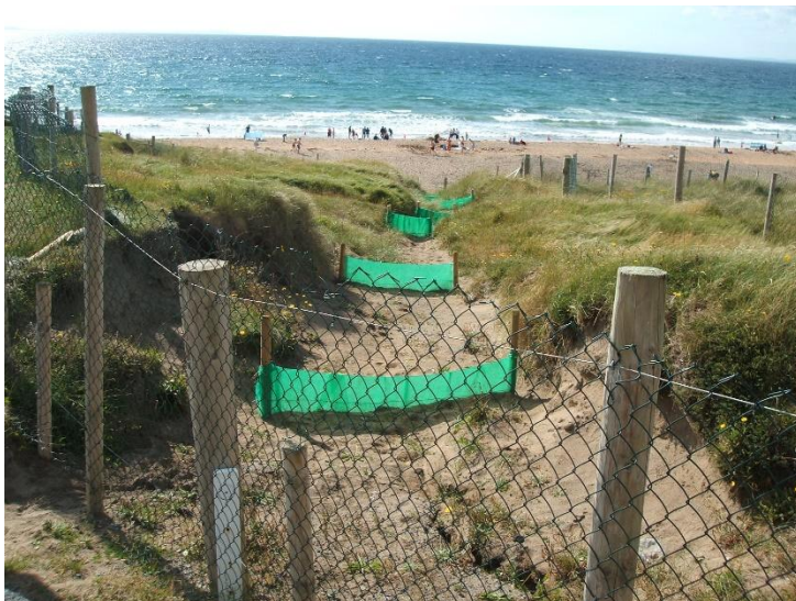
Photo 16: Sand trap fencing along gully at north end of dune (2005)
