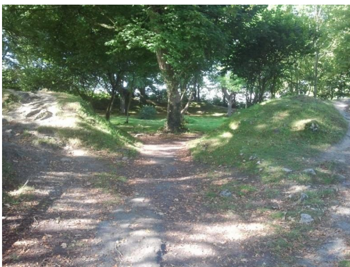
Photo 2 : Eroded entrance to the centre of An Rath
