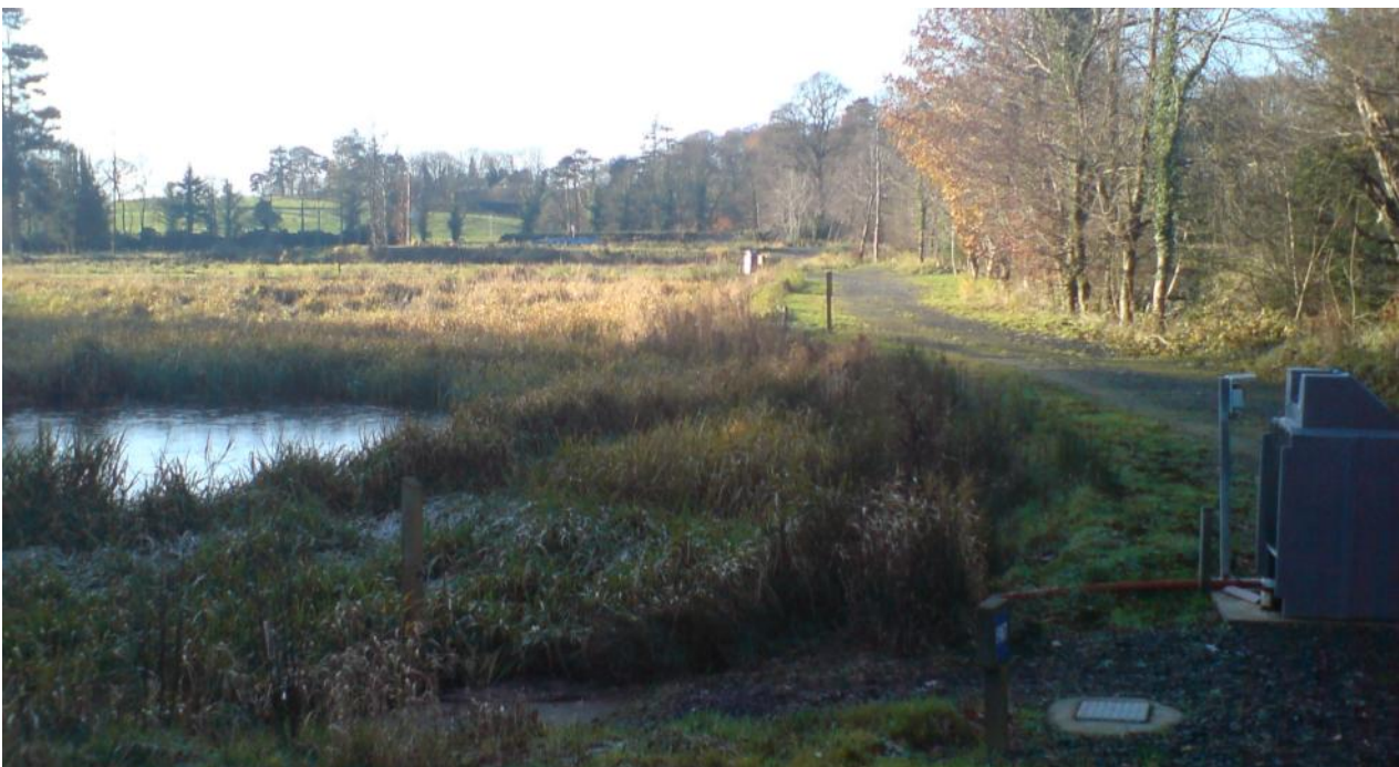
Glaslough Integrated Constructed Wetland, Pond 5. Photo by Pat Byrne
