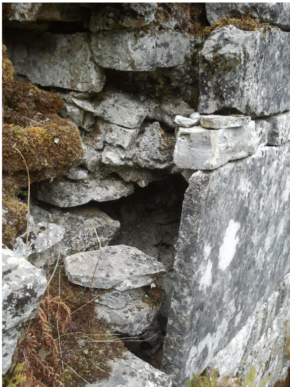
Photograph 17: Supporting flagstone on interior leaf of gable (August 2014)
