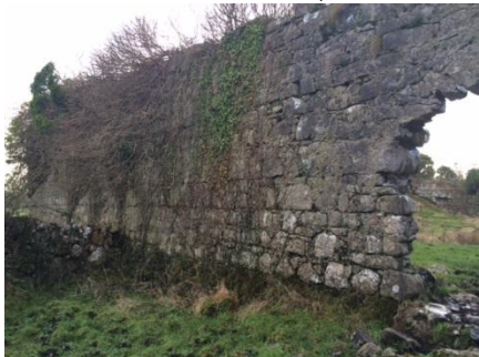
The northern exterior wall showing ivy growth
