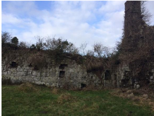
The interior western side of the building
